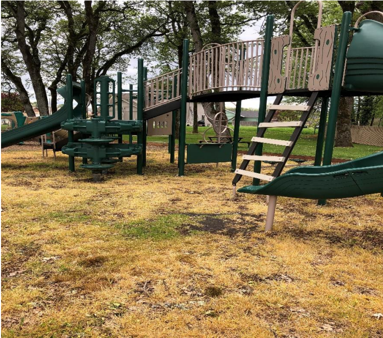
Exhibit B: Acorn Park – Maintenance needed to remove weeds and grass, to provide proper and adequate fall protection.
