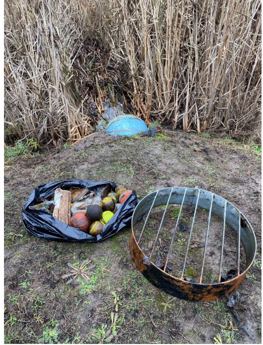
Debris and Grate Removed from Outfall
