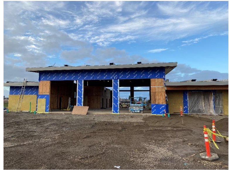
Figure 14: South exterior of station
