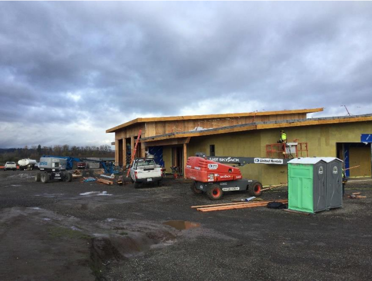
Figure 17: Looking northwest onto the south face of the building (11/04/2021)
