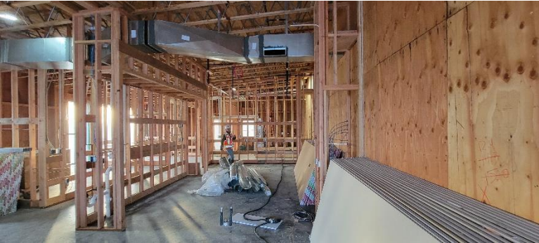
Figure 5: Looking west from the Dining Area into the Kitchen
