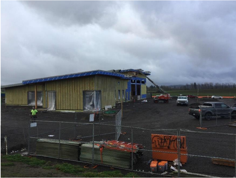
Figure 16: Looking southwest onto the north face of the building (12/08/2021)
