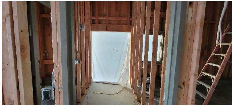
Figure 3: Looking west from the Lobby into the Apparatus Bay
