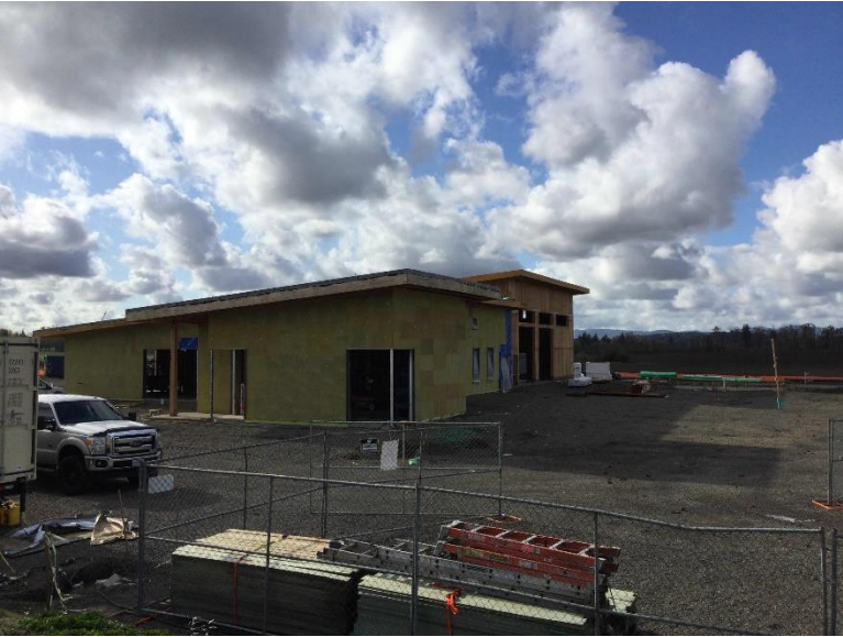
Figure 15: Looking southwest onto the north face of the building (11/05/2021)
