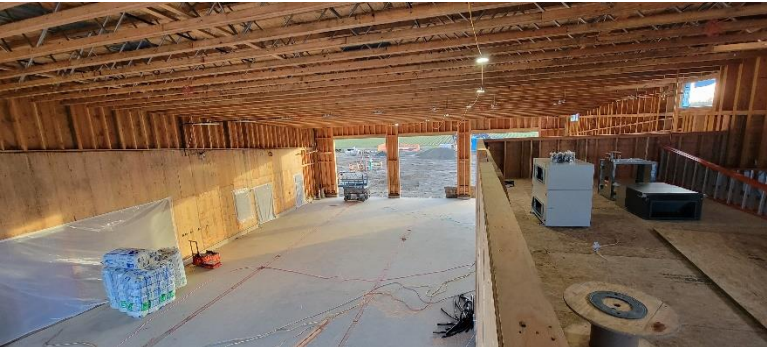
Figure 11: Looking south across the Apparatus Bay from the Mezzanine
