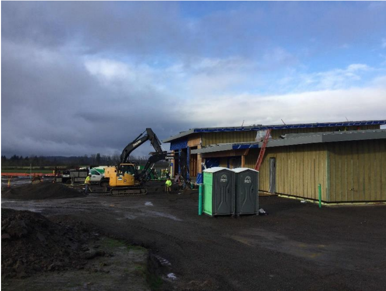
Figure 18: Looking northwest onto the north face of the building (12/08/2021)
