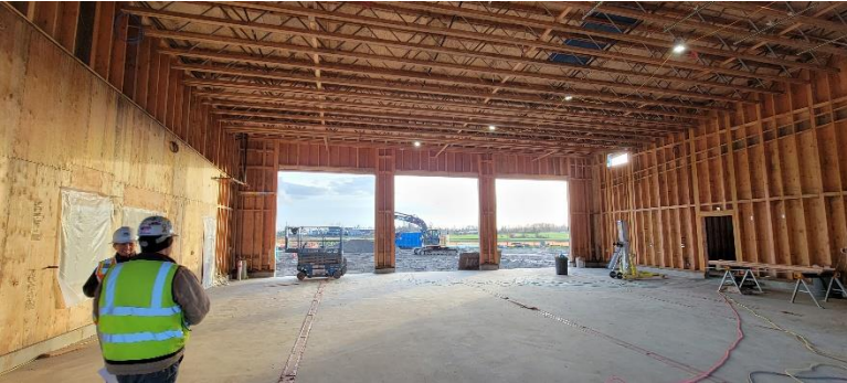
Figure 9: Looking south from the floor in the Apparatus Bay
