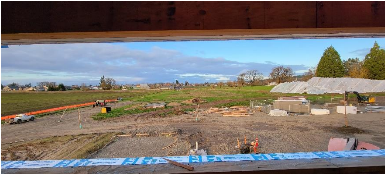
Figure 12: Looking north from the Mezzanine
