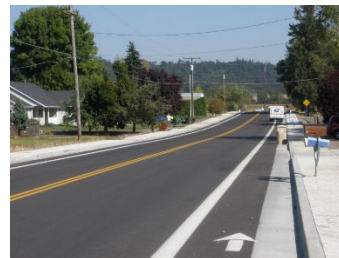
Alexander Drive (looking east) provides bicycle and pedestrian access to Millersburg City Park but lacks a safe pedestrian crossing
